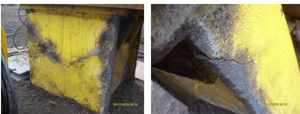
Fig.8. Cutting of damaged supports
