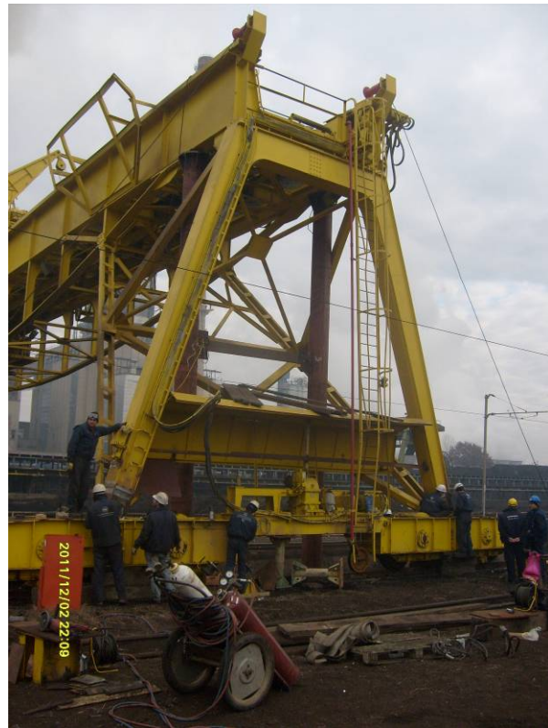
Fig.9. Preparation for welding
