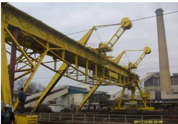
Fig.1. Coal-reloading bridge Metalna 300
