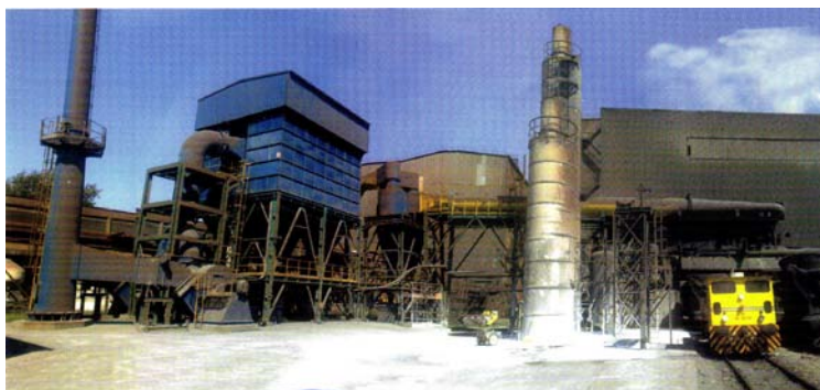
Figure 1. New facility for off gasses treatment in USS Serbia steel plant.
